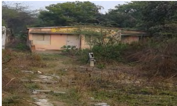
Before improvements, December 2014: ANM sub-center
